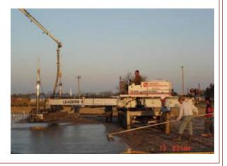
There are areas of the slab where plumbing prevents the leveling machine from being used and the laborers must finish those areas by hand.
